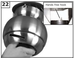
Hang fan from mounting bracket by the hands free hook into a closed hole on the edge of the Canopy. Note: For Canadian mounting refer to Step #10.
